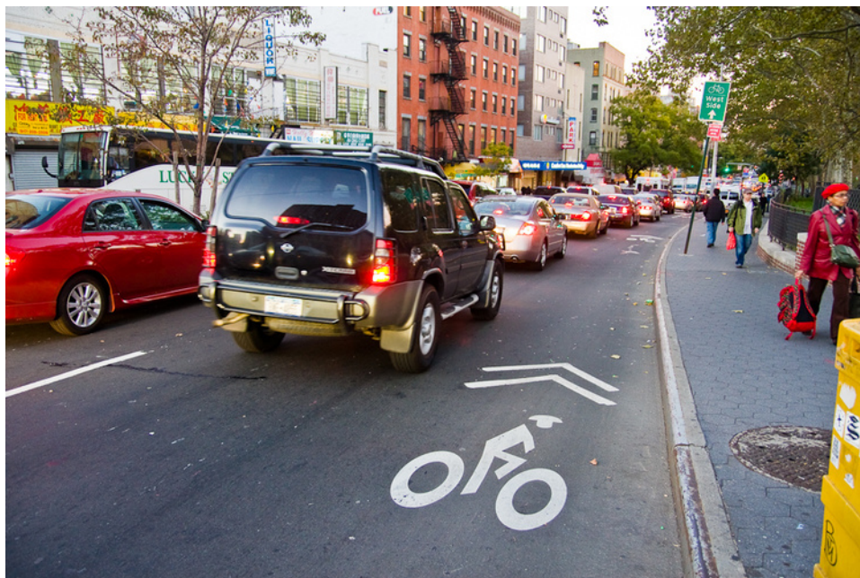
Figure 12. Sharrow, or shared lane marking
