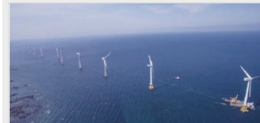
Tamra Offshore Wind Farm In Jeju Island(30MW)
