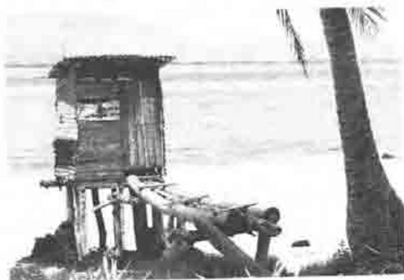
Manono Island. Although not common, over-the-sea toilets are still used in some locations. (photo: A.C. Robinson, reproduced courtesy of DLSE)
