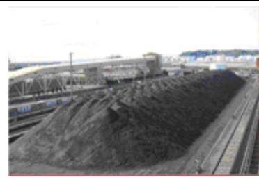
Coal stock yard Max capacity 165,000t 461m x 37m, 2pile
