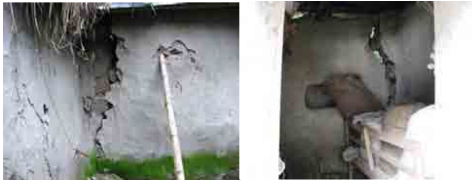
Fig. 18-1 Damages on houses in neighboring villages to Barapukuria coal mine
