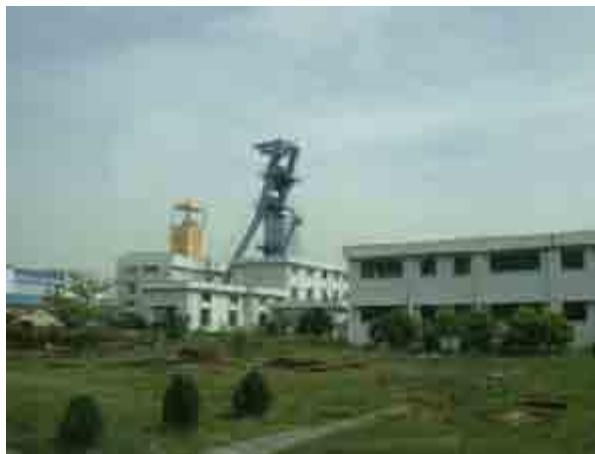
Fig. 4-7 Vertical shaft for material and workers and skip shaft for coal hoisting on rear side
