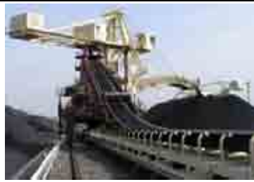
Stacker 2,000t/h Max piling height 9m
