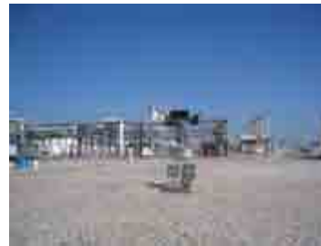
Bibiyana gas plant south area (2009/10/31)
