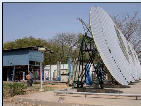
Figure 15 - Solar-Biomass Hybrid Cold Storage-cum-Power Generation system for Rural Applications installed at NISE, India
