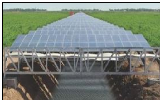
Figure 9 - 1 MWp Canal-top PV system installed over Narmada canal in Gujarat, India
