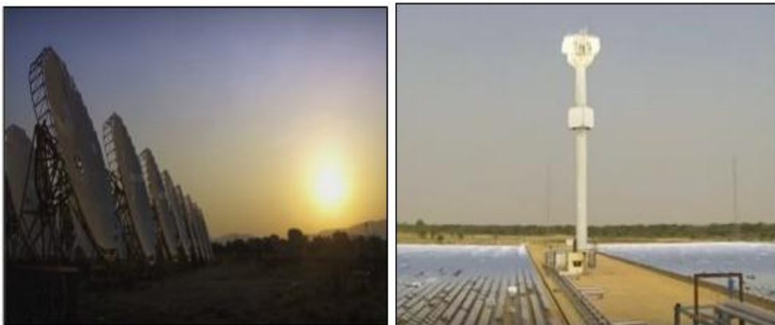
Figure 12 - Parabolic Dish System (left) & Central Receiver Tower (right)
