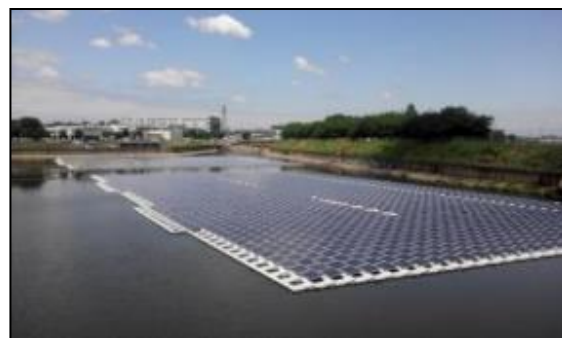
Figure 8 - A floating PV system of 1.15 MW capacity installed in Okegawa, Japan
