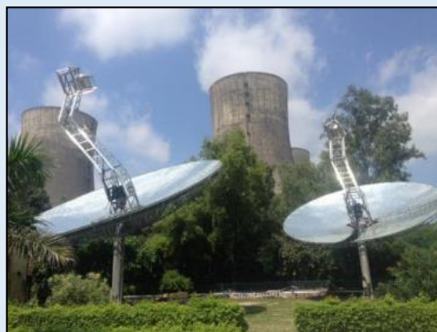
Figure 14 - Solar Thermal-LPG Hybrid Smart Cooking at a Power Plant Staff kitchen at NTPC- Dadri, India
